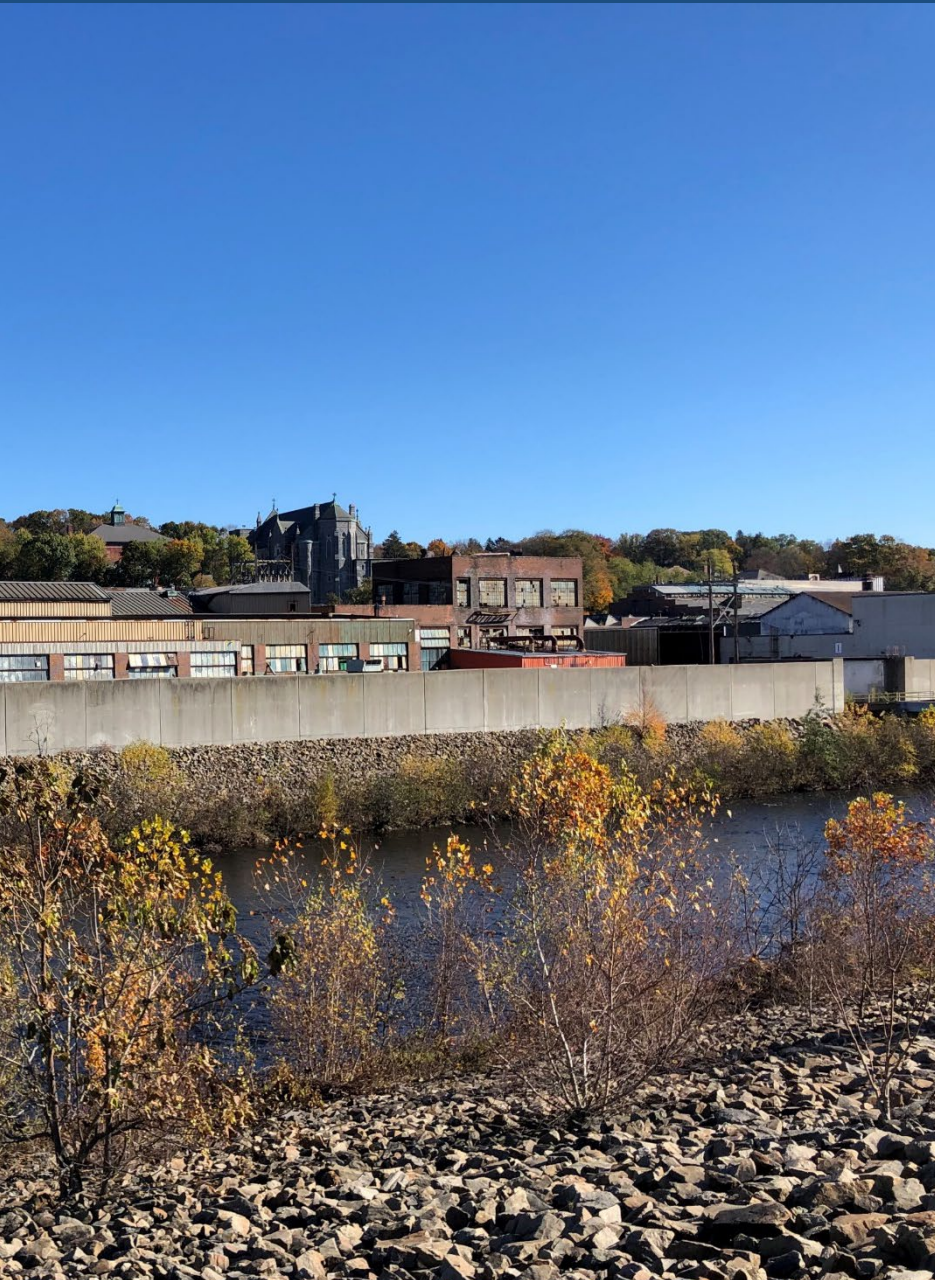
Photo of Flood Wall & Copper and Brass Facility Photo Credit: CIRCA
